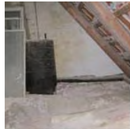
Gammel ekspansionstank.
